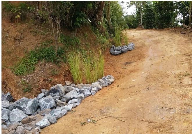
**Figure 51.** Example of check dams constructed by PDC on a dirt road network in Hacienda Candelaria located on the coffee region of Yauco Puerto Rico.
