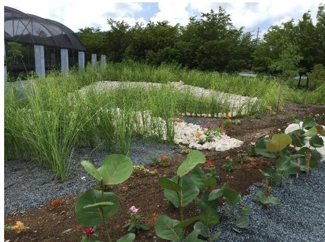
**Figure 43.** Example of a vegetated filter strip prepared by PDC personnel at the facilities of PDC in Yauco, PR. This strip helps to redirect and filter rainwater before arriving at the nearby river.
