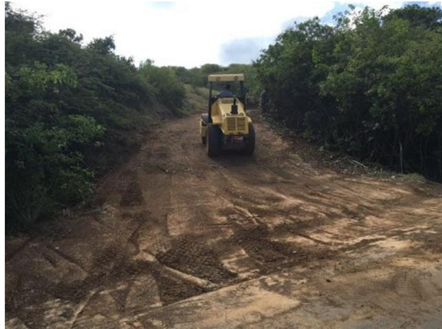
**Figure 50.** Example of regrading by PDC on a dirt road in Culebra, Puerto Rico.
