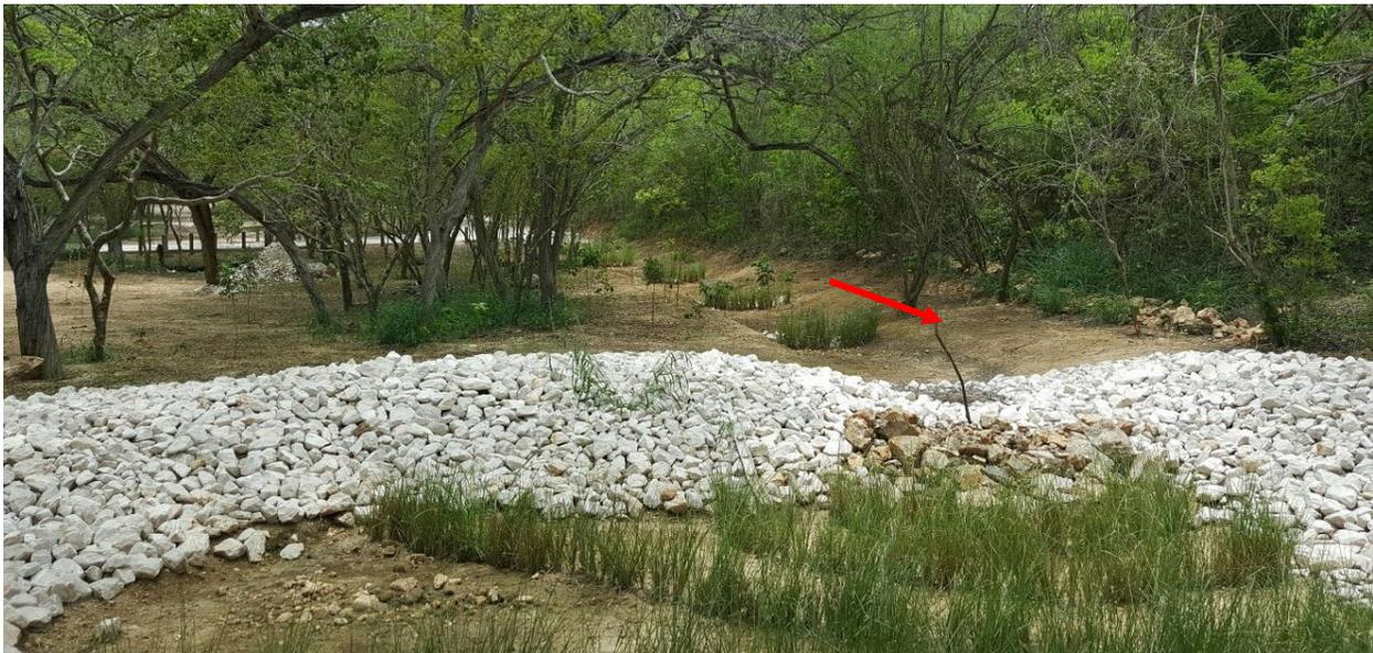
**Figure 40.** Example of a rain garden prepared by PDC personnel at Jaboncillo Beach, Guánica. The red arrow indicates the influx of water following a rain event. Water passes through the vegetation where it reduces its speed while nutrients and sediments are retained.
