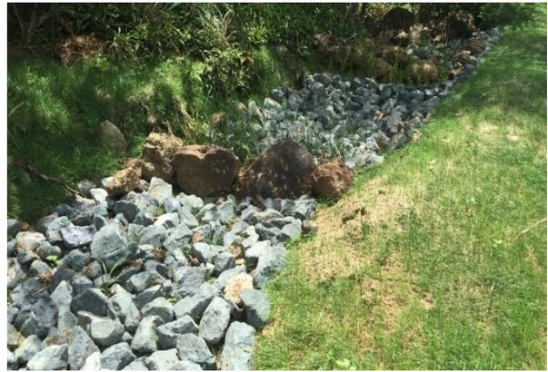
**Figure 42.** Example of a vegetated swale prepared by PDC personnel at Fulladosa, Culebra. In this design rocks were used along with the vegetation to create a channel.
