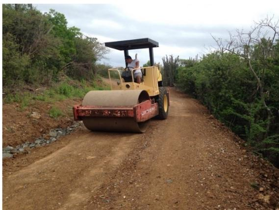
**Figure 48.** Example of dirt road stabilization techniques in Punta Soldado, Culebra, PR.
