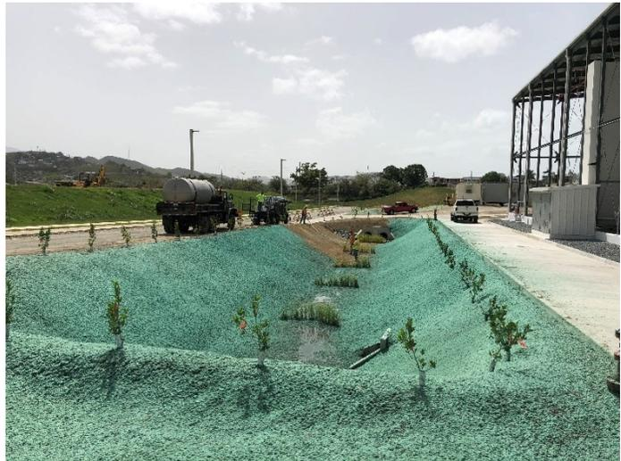
**Figure 46.** Example of hydroseeding application by PDC personnel at the facilities of Sartorius in Yauco, PR.
