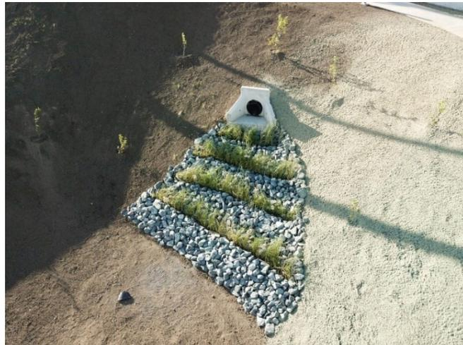
**Figure 47.** Example of a sediment trap technique implemented by PDC personnel at the facilities of Sartorius in Yauco, PR.
