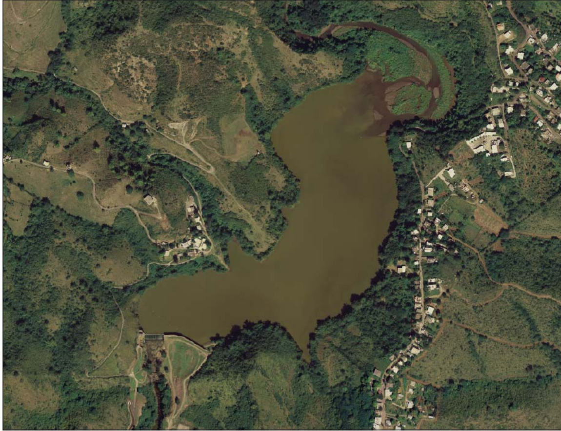
Figure 3. Snapshot of sediment accumulation and flow through Loco Reservoir.
